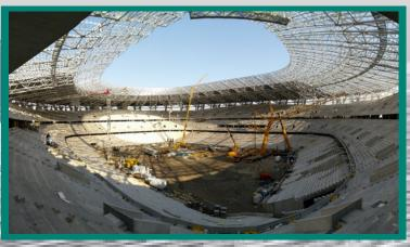
The stadium, totally rebuilt and completed in November 2019, sees the installation of Macrolux Rooflite greca 315/56.8 corrugated polycarbonate compact sheets in the translucent roof section, in a thickness of 2 mm, manufactured by Stabilit Suisse.
