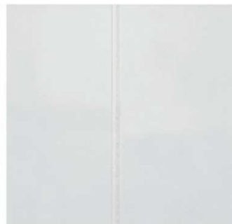
After 1/2 hour remove the tape leaving the sheet and the sealed joint uncovered.
