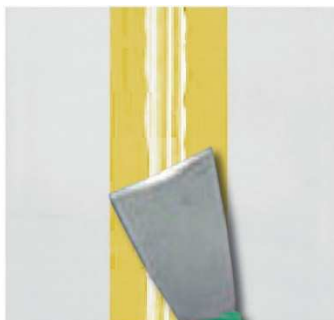
After 4 or 5 minutes, spread with a spatula to remove the excess of sealant.
