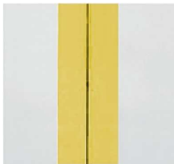
Protect the front of the sheets with adhesive tape to prevent staining.
